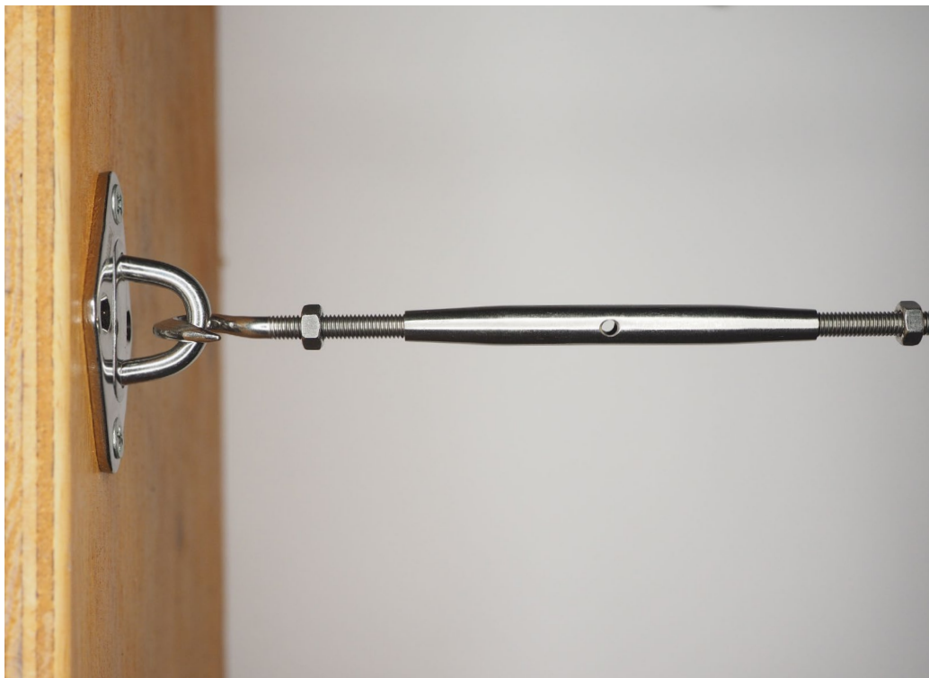
Fig 3.1 Reattach turnbuckles to each mounting device ensuring they are at their fully extended state as pictured.
