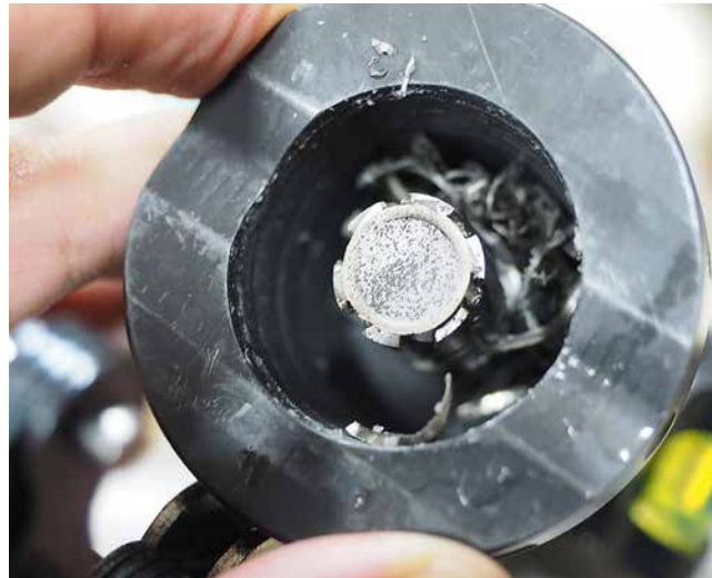
After drilling EACH hole, inspect the cutter assembly. Check for a slug and swarf build up (present in the above image)
